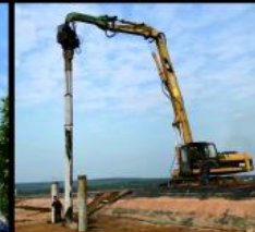
Pile driving arm
