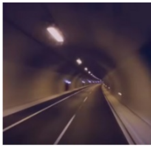
Highway construction tunnel
