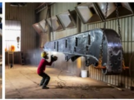
Spray painting Sandblasting and spray painting for anti-corrosion.
