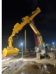
Cleaning and dredging
