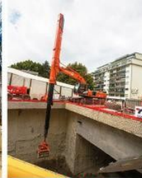
Deep pit work
