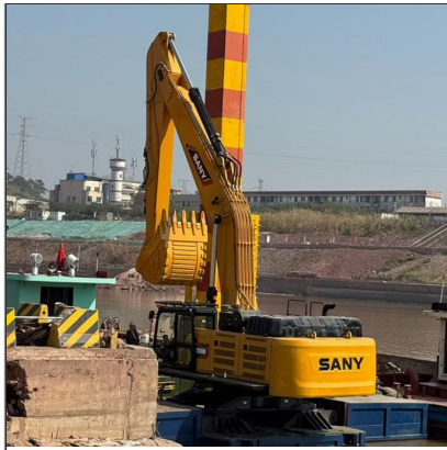
* Dredging * River Project
