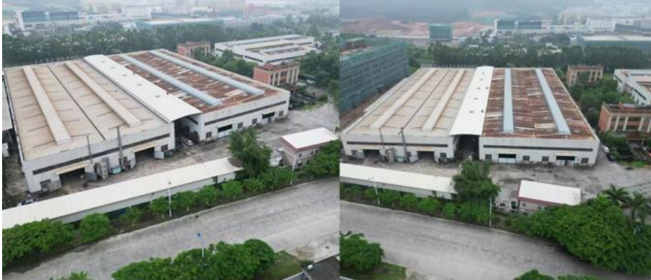
18000M 2 Steel Structure Workshop with Super Precision Machines
