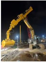
Cleaning and dredging
