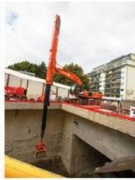
Deep pit work
