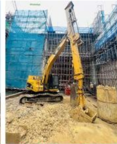
Bridge construction projects
