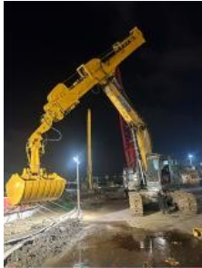
Cleaning and dredging
