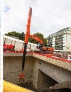
Deep pit work
