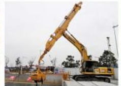
For unloading materials
