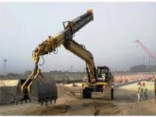
For Large-scale earthworks
