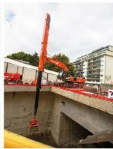
Deep pit work
