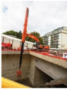
Deep pit work
