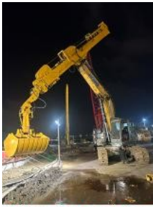
Cleaning and dredging
