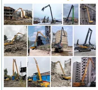
Excavator demolition arms operate effectively under various conditions, such as high-altitude demolitions, confined urban spaces, and during the dismantling of heavy industrial facilities. Their versatility allows them to tackle both broad and intricate demolition tasks efficiently.
