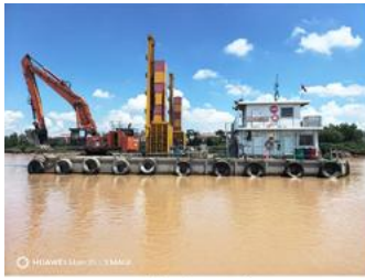
For canal cleaning
